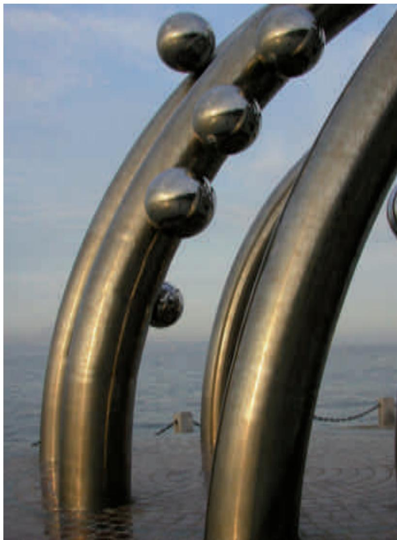
This sculpture right next to the ocean shows corrosion staining on type 304 stainless steel due to incorrect grade selection in a demanding environment.
